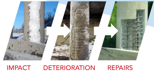
IMPACT DETERIORATION REPAIRS
